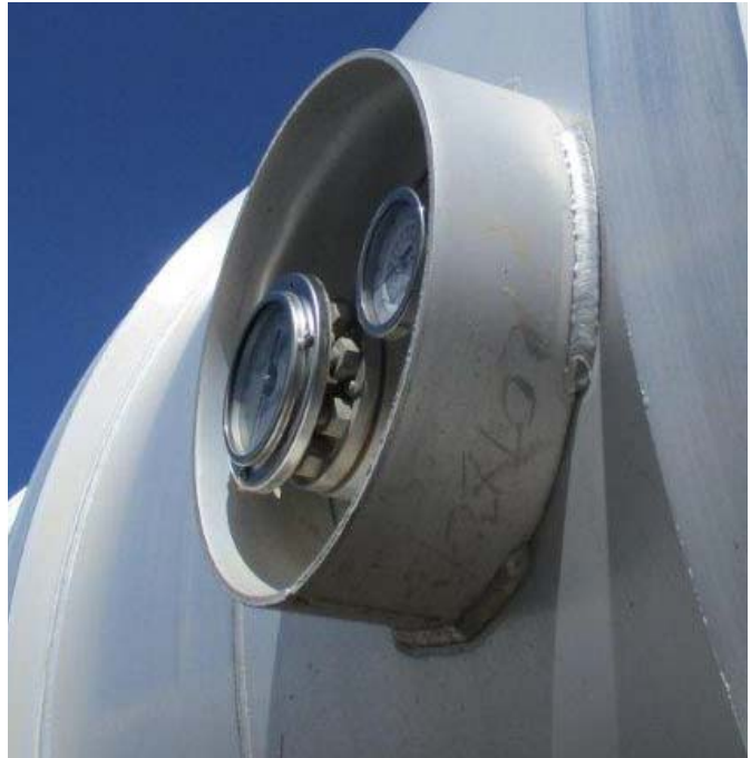
Example of Improper Pad
