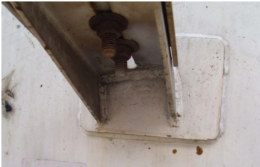
Example of Improper Pad
