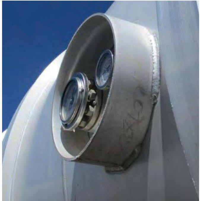
Example of Improper Pad
