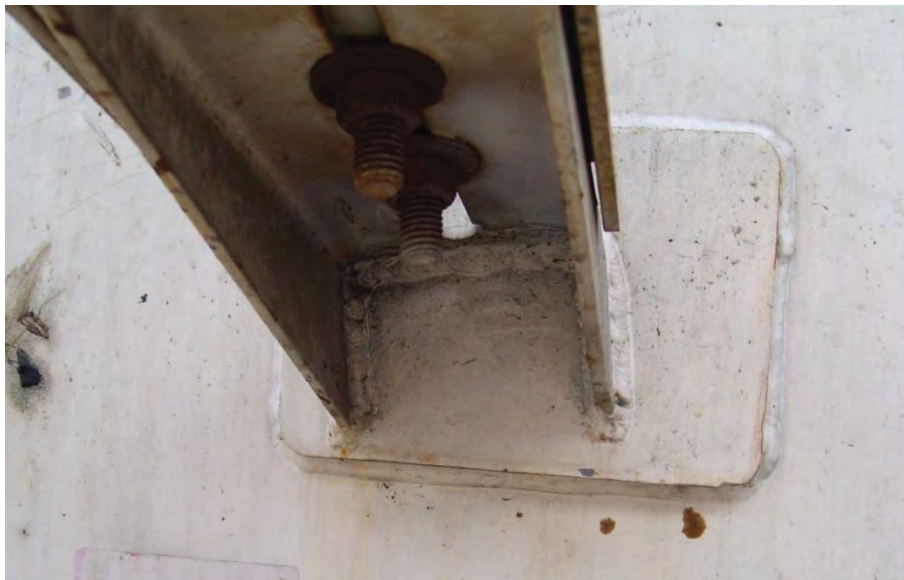
Example of Improper Pad
